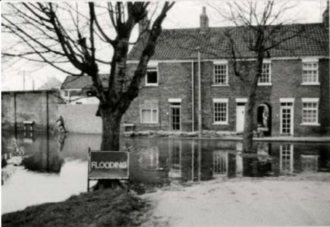
Flooding of Soutergate/Beck Hill, Feb 1980 (photo by Mr J. French)
